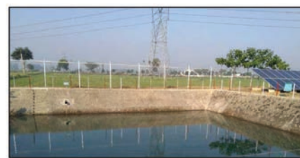
Figure 4. Community Water Storage Tank using solar power operations
