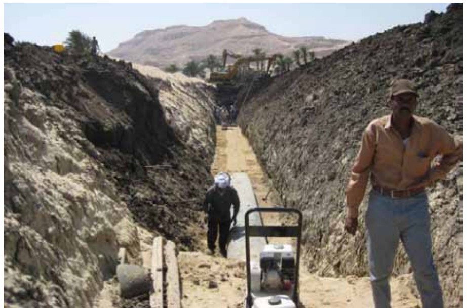
LAYING OF A MAIN COLLECTOR IN UPPER EGYPT
